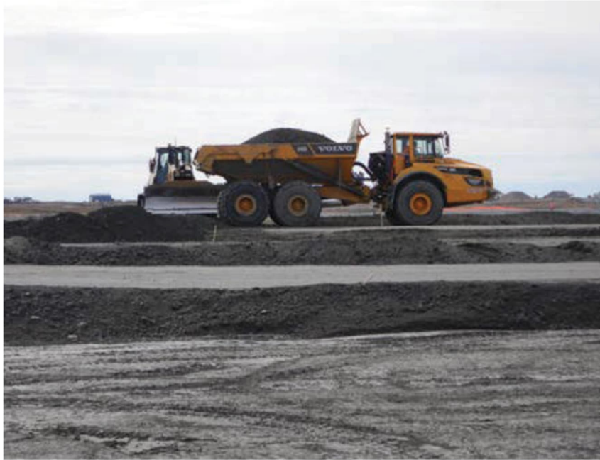
Figure 20-29 – Filtered Tailings Placement, Spreading and Compaction
