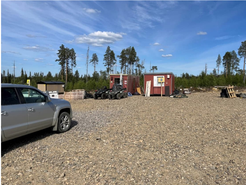
Figure 12-1 – Ikkari Project Site
